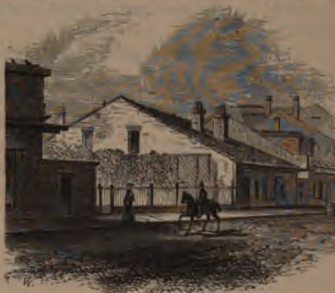
"Some aged private dwellings, rapidly decaying."
